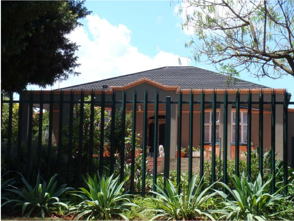
Typical house north of Goldman
