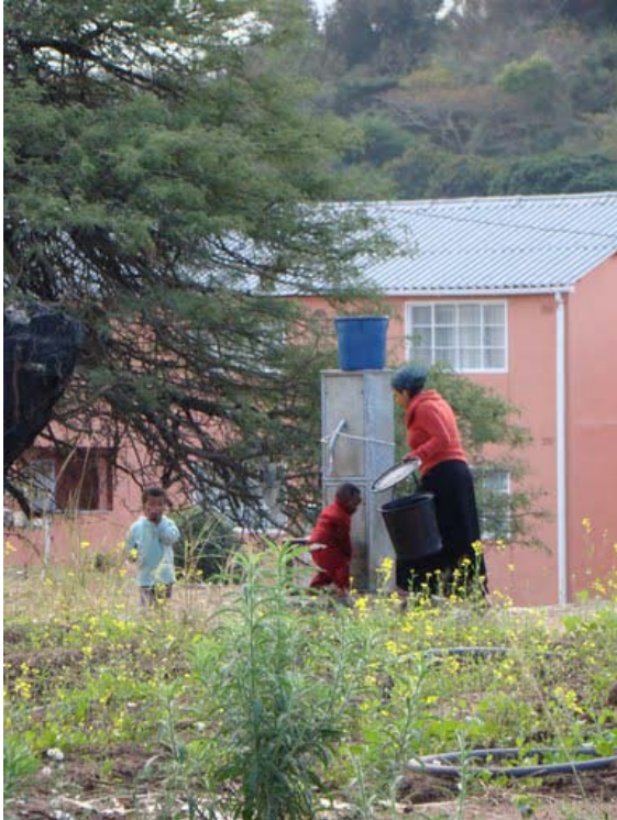
Left: Communal standpipe servicing Ekhupholeni informal settlement (Source: Amy Kracker, August 2009)
