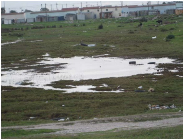
Detention Pond Collecting Water
