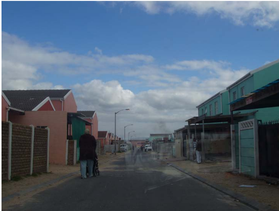
Cape Town Community Housing company homes
